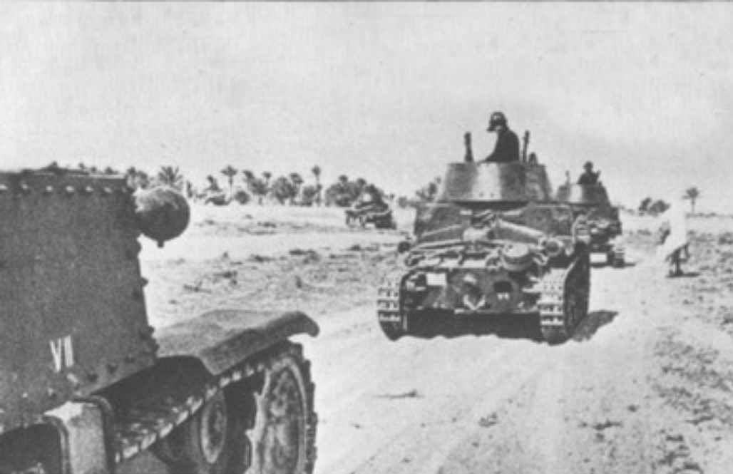
M 13-40s assigned to the VII (7th) Tank Battalion advance along a Libyan road in early 1941. A jack was placed on the aft port hull cover from hull 0752, while the spare road wheel was retained on the starboard side. This Battalion was assigned to the Ariete Armored Division, which saw extensive action in North Africa. (Cappellano)
