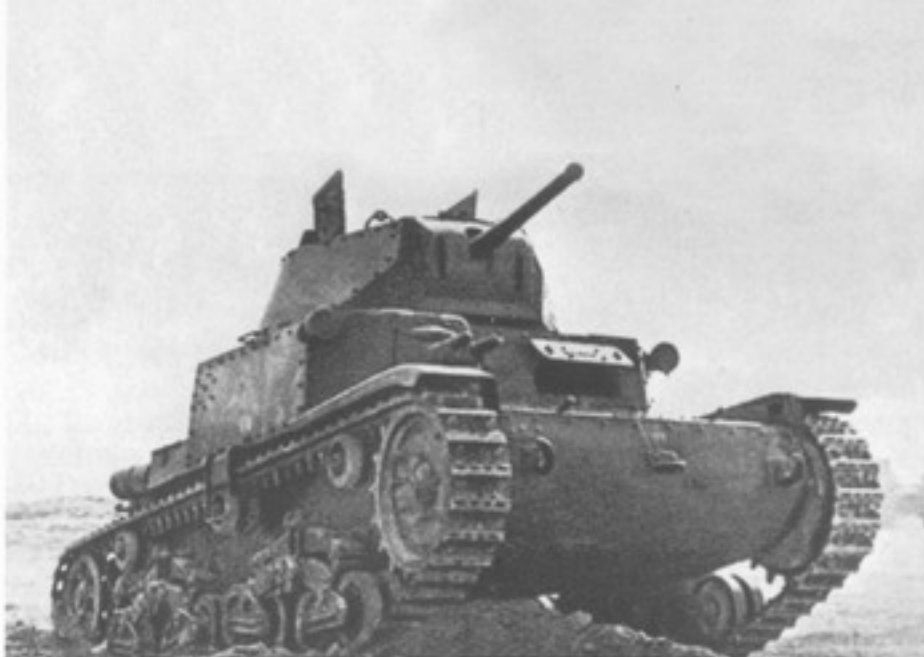
A VII Tank Battalion M 13-40 is perched on a slight rise in the desert in Cyrenalca, the eastern province of Libya. The tank was painted overall Gray-Green when it was sent from Italy to Libya in early 1941. The two-part turret roof hatch opened outward to allow the commander/gunner and the loader access to and from the turret. (Cappellano)
