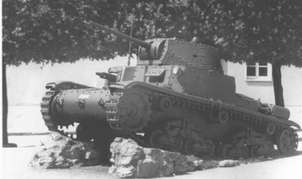
The M 15-42 was the final M ( Medio ; medium) tank developed for the Regio Esercito . This vehicle featured a 47mm Ansaldo L40 gun, 45mm front armor, and a 190 HP Fiat SPA 15T gasoline engine. The M 15-42 just entered Regio Esercito service when Italy reached an Armistice with the Allies on 3 September 1943. The radio antenna could be raised or lowered from inside the vehicle. This particular M 15-42 was repainted overall Olive Drab (FS34087) and served with the Italian Army after World War Two.
