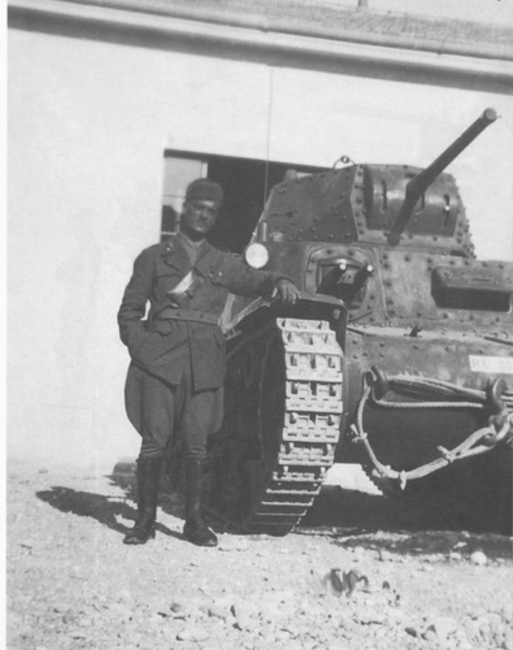
A tank officer stands beside an M 13-40 (R o E o 3052) during his training period. Armored personnel wore red and sky blue collar patches on their gray-green uniforms. The Royal Italian Army's vehicle registration number was only displayed on a stamped plate on the tank's left rear before mid-1941, when this number was also painted on the front hull. The registration was in red lettering and black numbers on a white background. (Palma)
